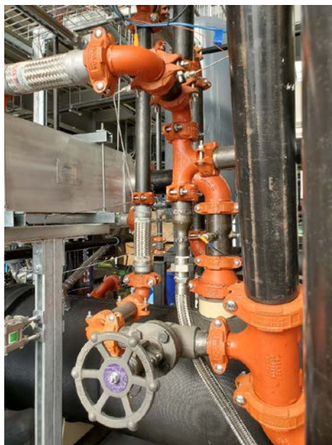
Figure B-3 Test facility turbine bypass loop
